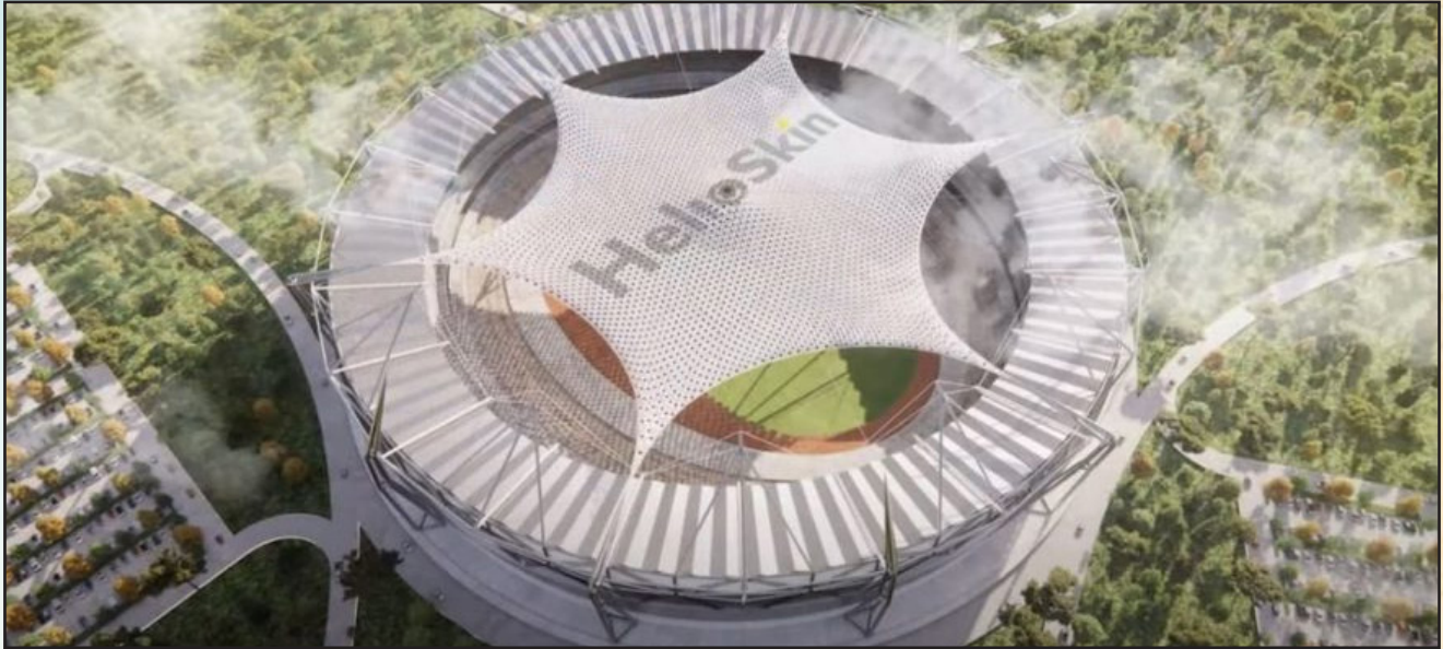
The HelioSkin above a stadium will not only protect from sunlight but will also capture photons to generate electricity for lighting the stadium.
