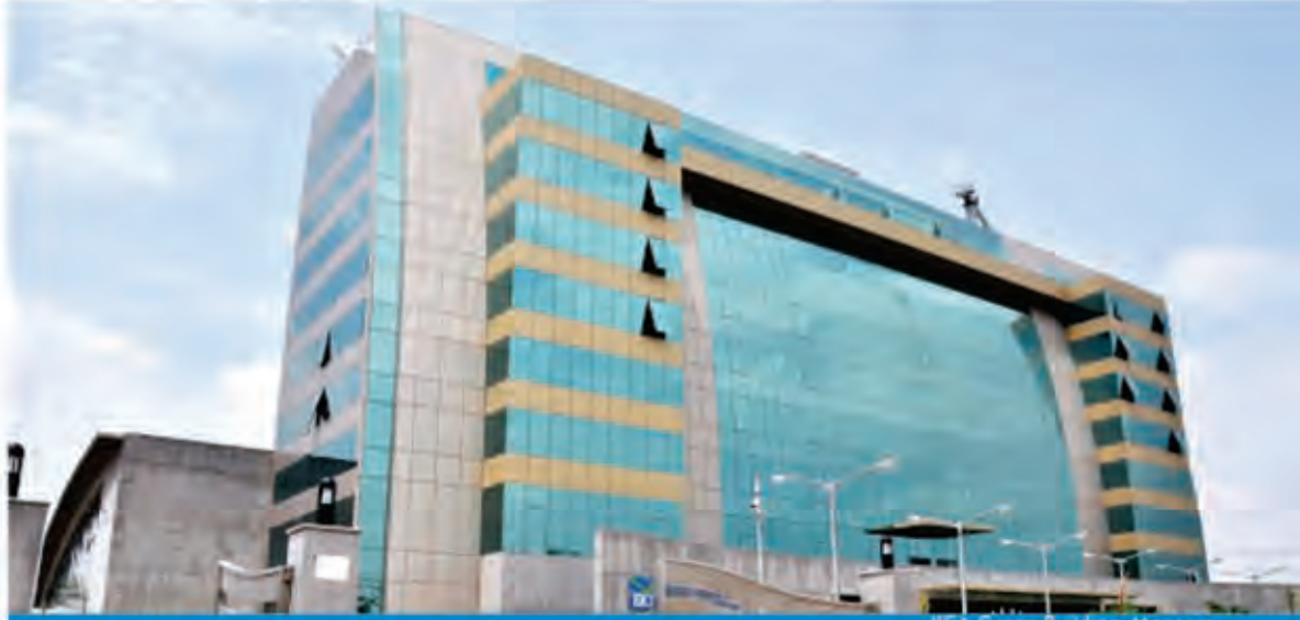
IICA Green Building, Manesar
