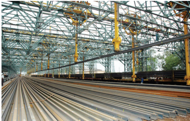
Automated Rail Loading Facility
