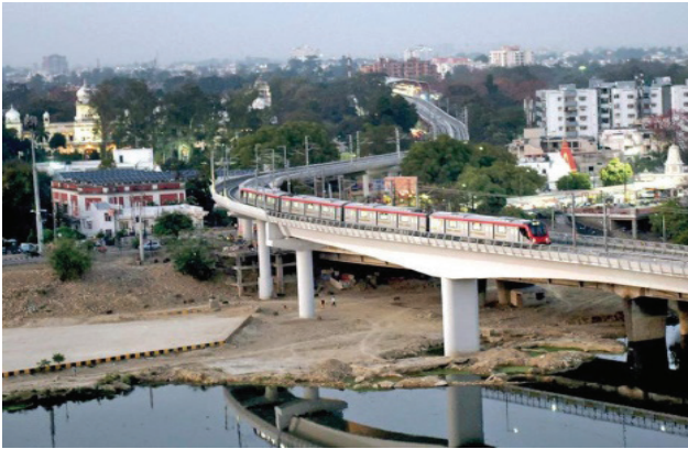
Metro Rail Projects
