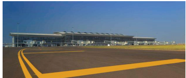
Hyderabad International Airport
