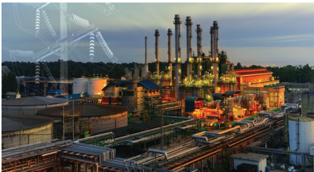
Nabinagar Super Thermal Power Project
